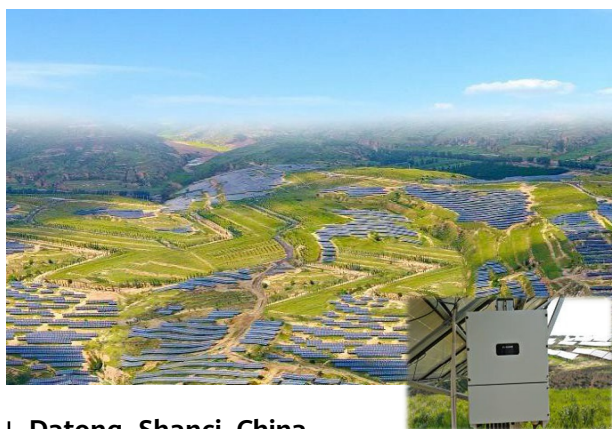
Datong, Shanci, China Mountain-mounted Smart PV Plant Capacity: 100 MW Inverter Model: SUN2000-40KTL
