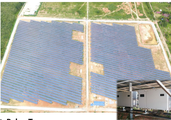
Paka, Terengganu Ground-mounted Smart PV Plant Capacity: 30 MW Inverter Model: SUN2000-90KTL-H1
