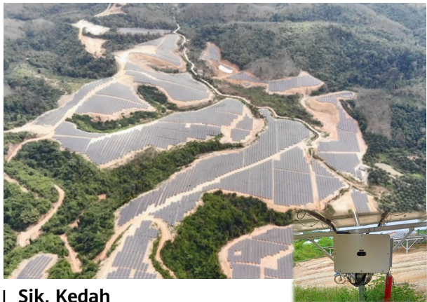
Sik, Kedah Ground-mounted Smart PV Plant Capacity: 30 MW Inverter Model: SUN2000-185KTL-H1
