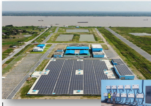
Vietnam Capacity: 760kWp Inverter Model: SUN2000-36KTL
