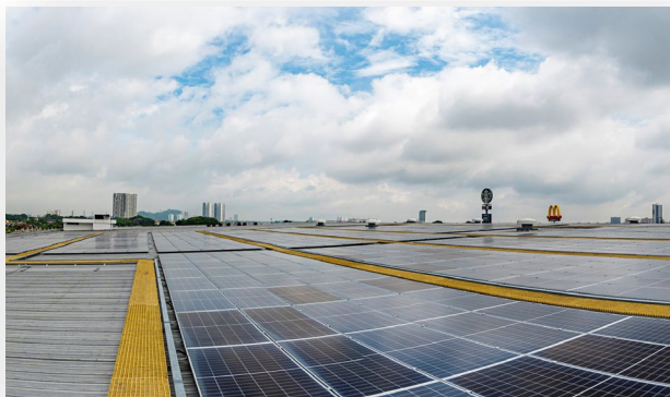
Malaysia Capacity: 636 kWac Inverter Model: SUN2000-100KTL-M1 SUN2000-36KTL-M3
