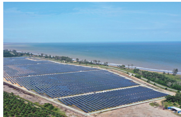
PV Park Pekan, Pahang GPS Tracker PV Plant in Malaysia Capacity: 45 MW Inverter Model: SUN2000-90KTL-H2
