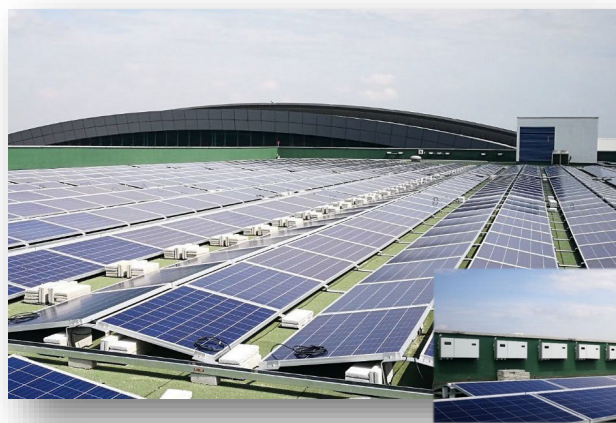
Singapore Capacity: 2.8 MWp Inverter Model: SUN2000-36KTL
