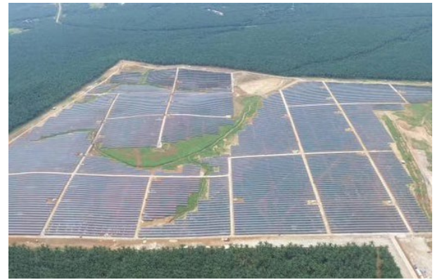
Kuala Ketil, Kedah GPS Tracker PV Plant in Malaysia Capacity: 50 MW Inverter Model: SUN2000-42KTL
