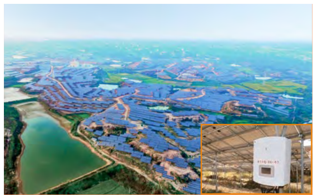
Zhejiang Longyou Agricultural-photovoltaic hybrid PV plant 25MW
