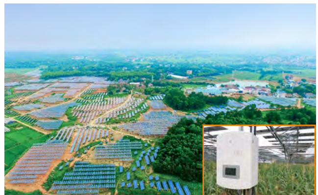
Quzhou Qinghu Agricultural-photovoltaic hybrid PV plant 20MW
