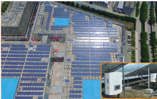
Ninghai AB hall, modern home plaza 1.53MW
