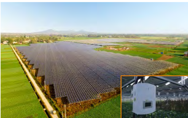
Hubei Guanyin Agricultural-photovoltaic hybrid PV plant 20MW
